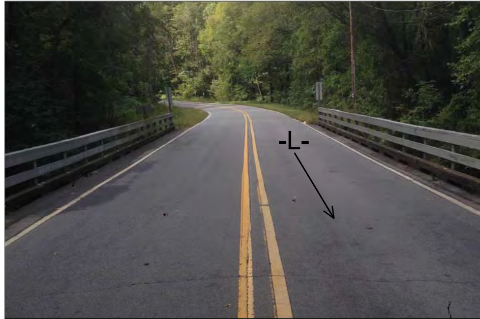
LOOKING DOWNSTATION ALONG -L- FROM NEAR END BENT TWO
