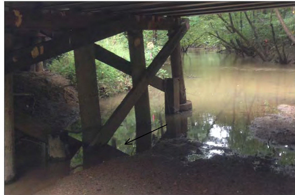
EXISTING INTERIOR BENT, LOOKING UPSTREAM
