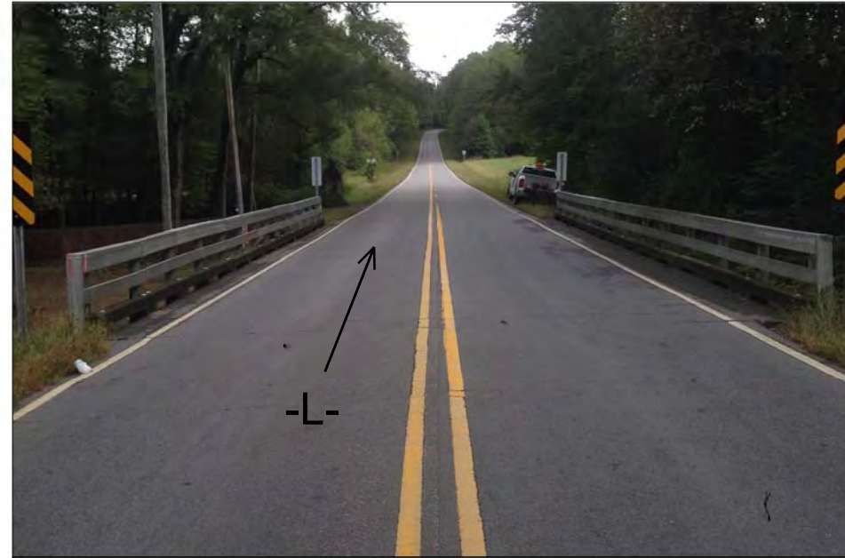
LOOKING UPSTATION ALONG -L- FROM NEAR END BENT ONE
