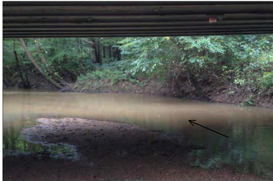
LOOKING DOWNSTREAM FROM UNDERNEATH BRIDGE
